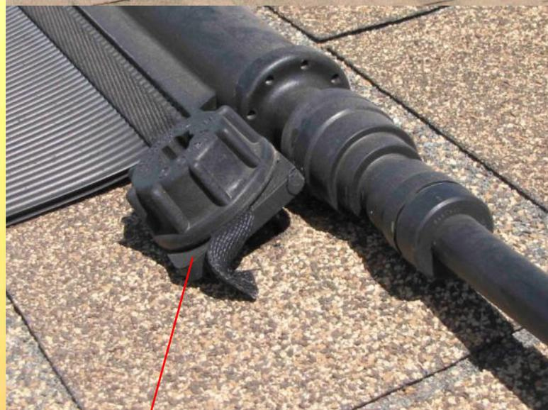
Tie-down tearing out of roof
