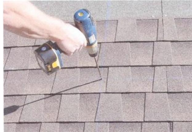
**2. Drill 1/4" pilot hole for lag bolt**
