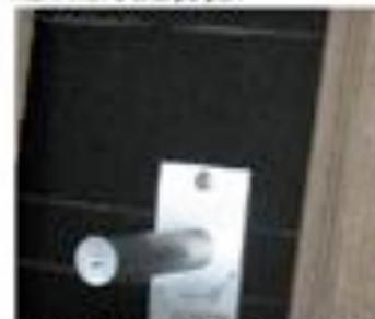
Drill 1/4" pilot holes for 2 each lag bolts. Drive lags into holes until secure
