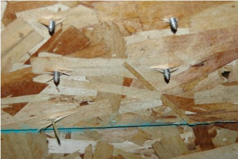
Lag bolts into the deck must go into **plywood** thicker than 1/2"
