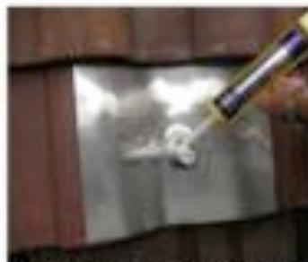
Install sealant around cone to post
