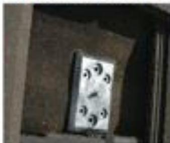
Use the Mounting Base as a template to mark the drilling of the 4 each 1/4" holes. Use a screw driver to break out the sealed portion.
