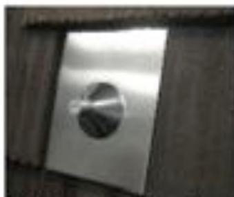
Apply a bead of sealant to post - flashing connection
