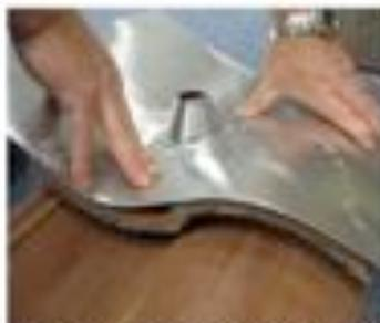
Place Aluminum Flashing into position over post and bend to the contour of tiles
