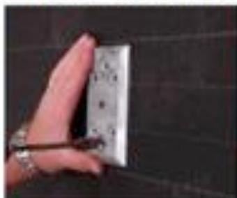
Use the Mounting Base as a template to mark the drilling of the top and bottom holes.
