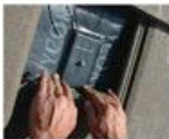
Apply peel and stick flashing over mount and up and under paper \*
