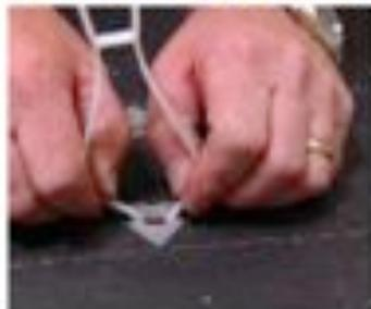
Remove Plate, drill 3/4" hole through deck. Insert toggler bolts per Toggles Instructions.
