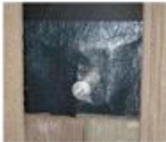
Re-install post onto stud. Make sure peel and stick slides under existing building paper
