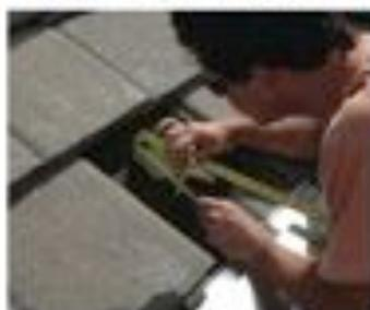
Remove Tile at location of Mount. Measure up 6 5/8" to center of mount. Mark paper, then measure 5 1/2" from exposed edge of adjoining right tile to center of mount, and mark paper.
