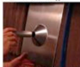
Insert post through flashing and secure to base threads.
