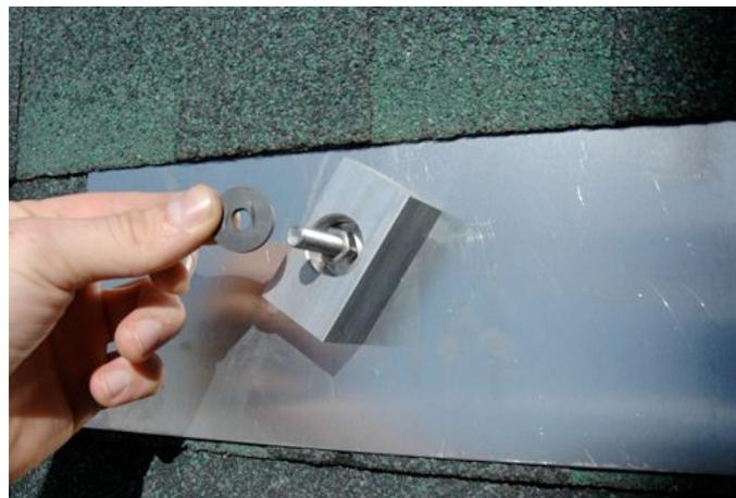
**6. Add EPDM rubber gasket to seal block**
