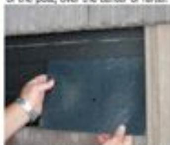
Remove post from plate, install "peel and stick flashing" over plate with stud protruding through hole
