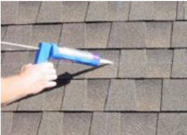
**3. Add roof sealant to pilot hole**
